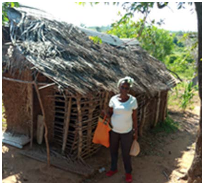
Over 90% of houses at the site are constructed with poles
