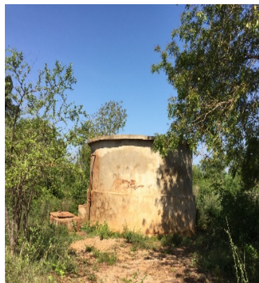
e) Water tank
