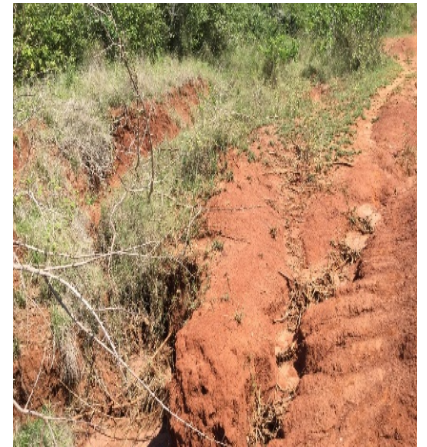
c) gully erosion
